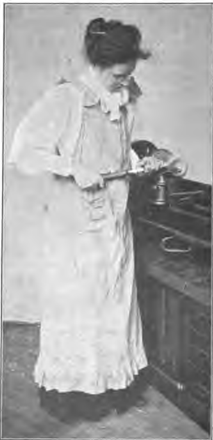
Fig. 187. Turning the Bead on the Cover.
